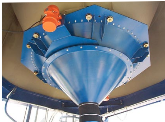
Bin Activator for lime discharging in a waste water treatment plant in Tennessee (USA)
