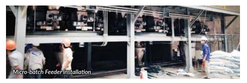
three RVS blow-through rotary feeders, twelve GT pipe couplings, four ILT level indicators, one WAMFLO® dust collector, one RVR drop-through rotary valve, four EXTRACURVE® wide radius pipe elbows, as well as four OT-type OLI® pneumatic vibrators. The systems have been successfully operating since the beginning of 2017.
