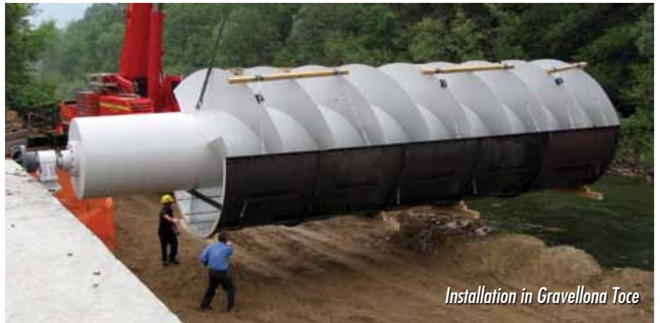
parallel the three screws bridge a drop of three metres reaching a nominal flow rate of 15 cubic metres per second. The total power generated amounts to 400
