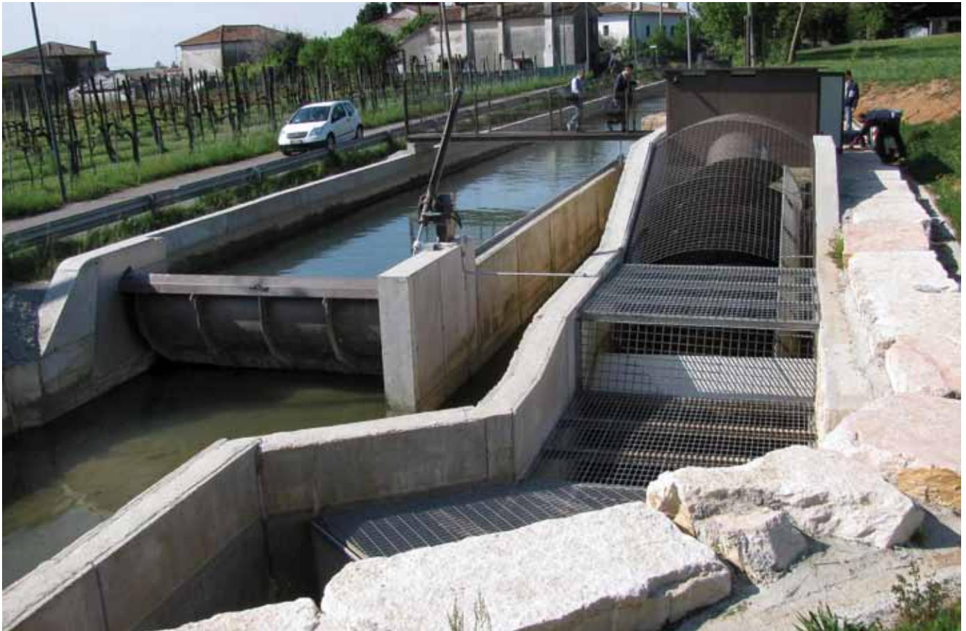
Left to right: original watercourse with big fan gate, small by-pass channel for water life preservation, hydrodynamic screw PAE
