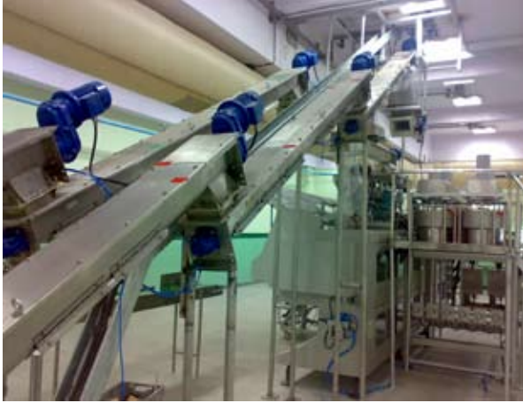
Trough Screw Conveyors in Unilever Factory in Nashik, India
