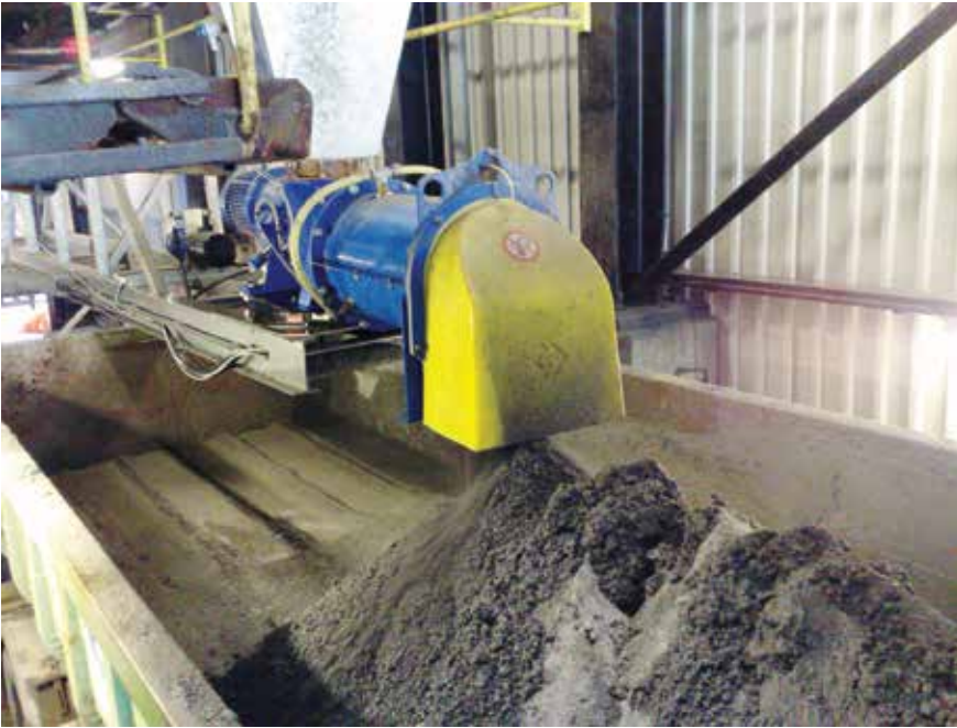
DUSTFIX® in operation for fly-ash disposal in a power plant in the Netherlands
