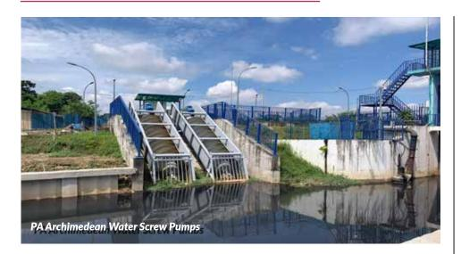
few kilometres southwest of the Malaysian capital Kuala Lumpur lies the small village of Bukit Lanchong, where WAM Malaysia in 2018 supplied two RONCUZZI® screw pumps with an external diameter of 1,900 mm to the JPS Department of Irrigation and Drainage. The Archimedean Screw Pumps are installed at the mouth of a small tributary of the Klang River to prevent flooding in bad weather conditions. The pumps are controlled by a level indicator and only operate during heavy rainfall.
