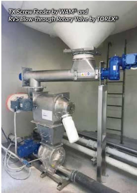
TX Screw Feeder by WAM® and RVS Blow-through Rotary Valve by TOREX®
