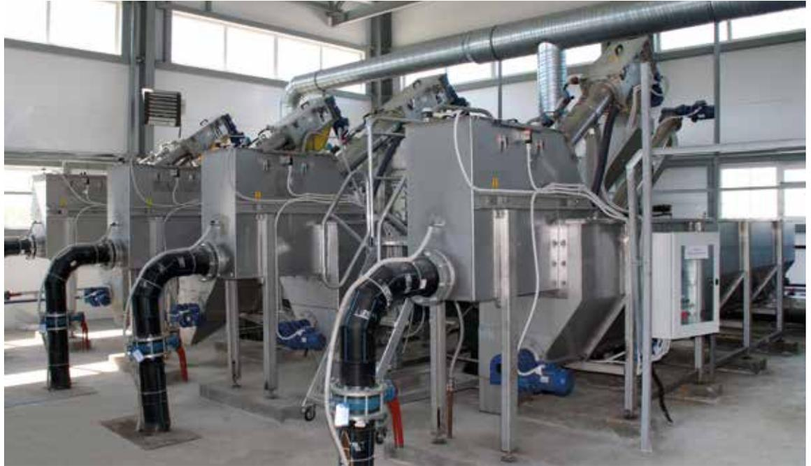
Each compact pre-treatment plant has a capacity of up to 30 litres per second and offers the operator optimum efficiency in mechanical pre-treatment and grit separation, which greatly ben-
