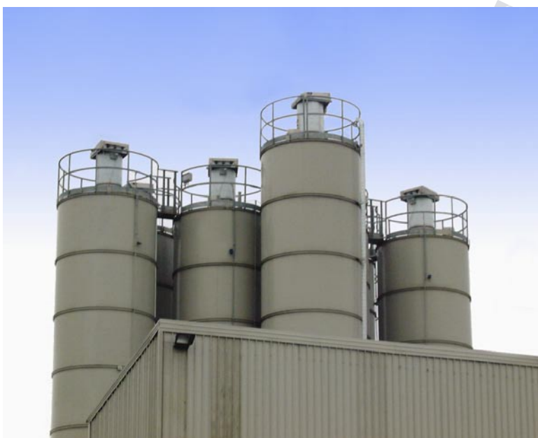
SILOTOP® Venting Filters installed on top of each silo in a concrete plant
